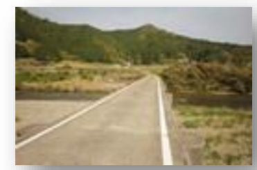
③ Nagano bridge
