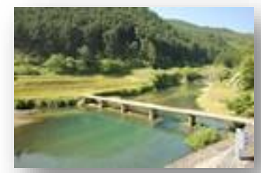
① Takahi bridge
